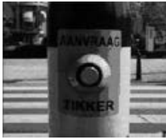
Fig. 6. Unclassified. In order to help the blind cross over, 'tickers' have been installed at zebra crossings, giving sonic cues to the state of the traffic lights. The sound sometimes lead to complaints from people who lived next to them, which, in turn, led to a most curious design solution: the ticking information has to be requested by pressing a button. How will the blind person find the button, or its function, the first time he or she comes here?
