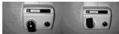
Fig. 5. Freedom. This hot air blower's nozzle can be directed down to dry your hands, or up to dry your hairs. How do you see that you can turn it? A sign 'turn here to make the machine blow up in your face' might at least amuse native speakers of English...
