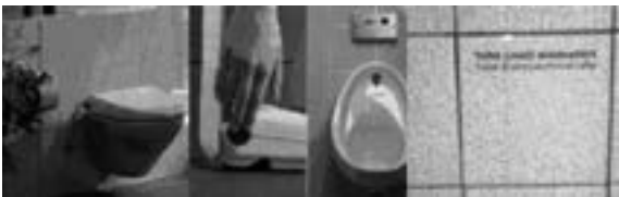
Fig. 2. Discreteness. Left: This toilet design has the flush button elegantly incorporated in its shape, so that it looks as a hinge, and finding the flush becomes a possibly embarrassing puzzle. Right: Public toilets show evolutionary stages due to the introduction of body proximity sensors. Some sensors look like buttons or ornaments, and don't express their sensing activity. After these sensors were introduced, signs were needed to tell people they didn't have to flush. Recently, we see the opposite: in some places where there are buttons, these look so similar to sensors, that signs are added that users had to 'please flush manually'.
