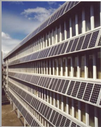
40 kWp PV Façade Northumberland Building
