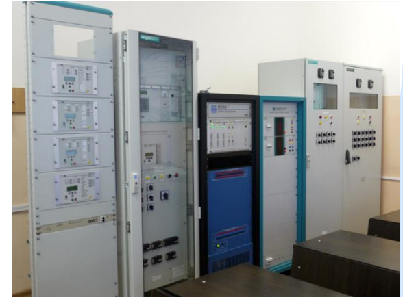
Relay protection and electric power system's automation laboratory
